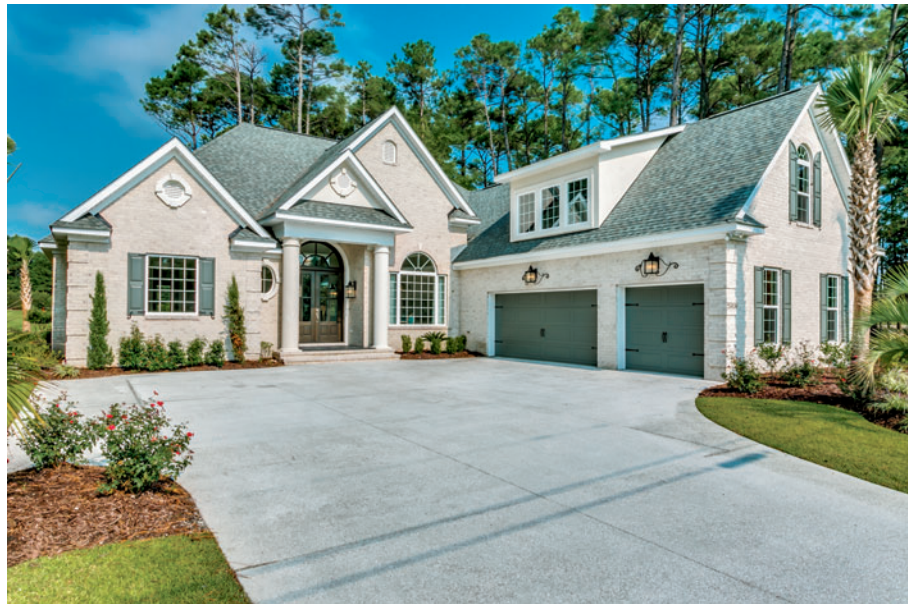
The Nations Homes II ‘Pine Lakes’ model. Homes built on your lot or existing lot start in the high 200’s.
